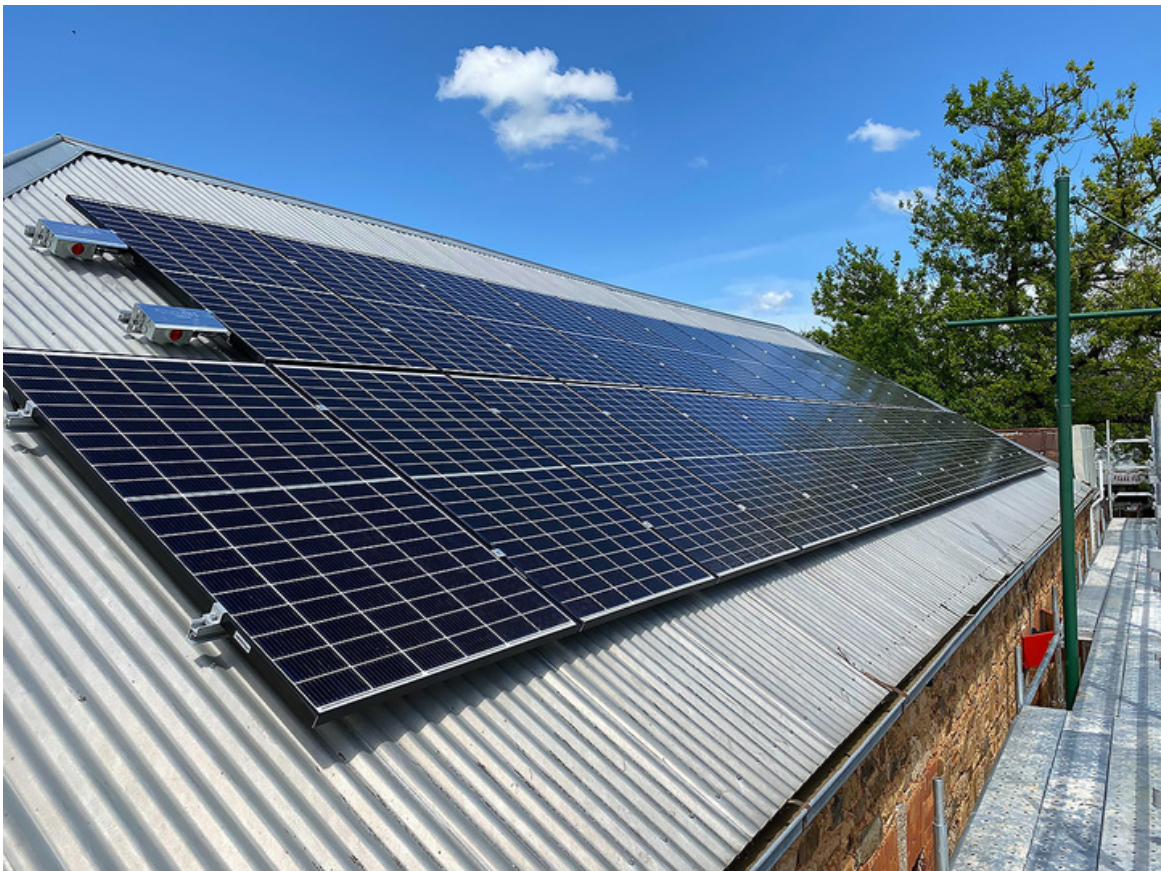
Solar installation on the Yack Post Office. Photo: Luke Fraser, Solar Integrity
