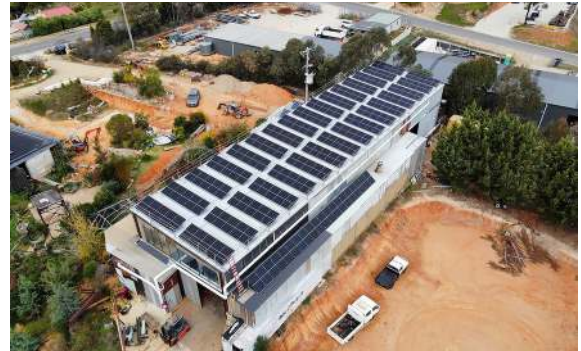
The 65 kW of solar panels on the roof of the old sawmill that are part of the Yack01 community battery installation.
