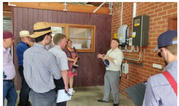
The existing 6 kW of solar panels and 13 kWh battery at the Yack CFA station will be backed up by a generator for emergencies. Matthew Charles-Jones showing the CFA clean energy installation to the Victorian government climate change enquiry earlier this year.
