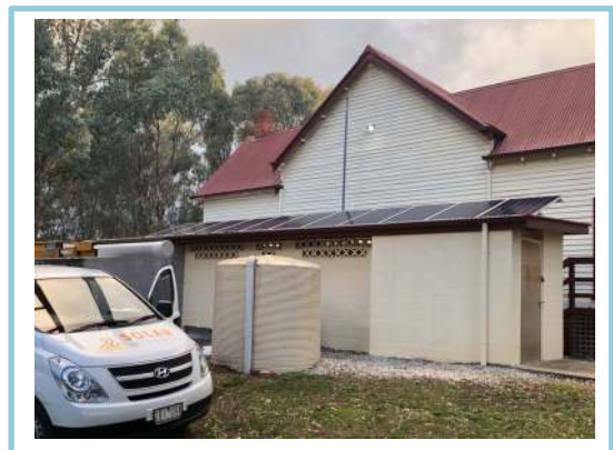
Osbornes Flat Hall during the recent installation of its new solar system
